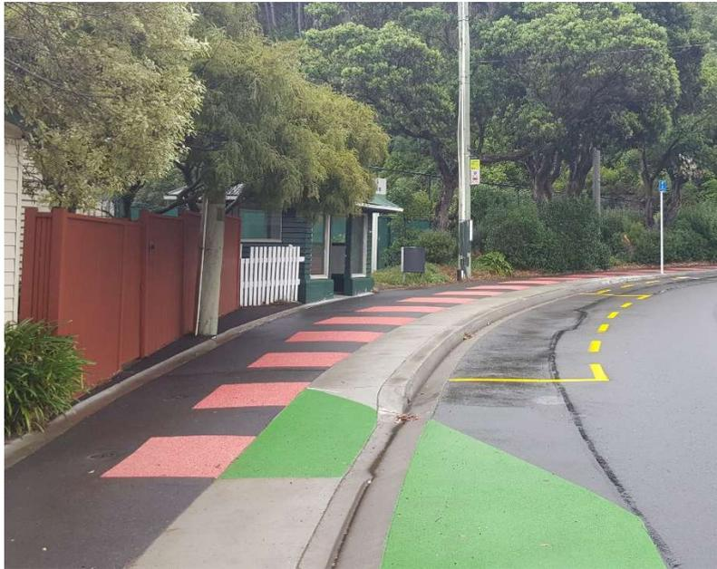
Cycle lane diverts onto footpath and passes between bus shelter and bus bay. Shared zone for cyclists and pedestrians is denoted by red stripes. A white concrete strip provides a boarding and alighting area for passengers. Site is on an uphill gradient.
