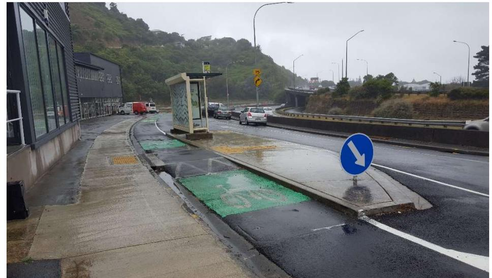
Cycle lane passes behind bus shelter. Pedestrian crossing to bus stop island is marked by a raised section of the cycle lane and tactile paving. Inbound. Daily boardings: 27, alightings: 11, total: 38
